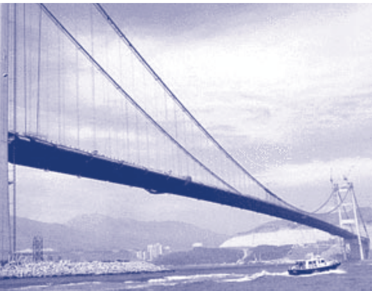
The Tsing Ma Bridge links Tsing Yi to Ma Wan, China. Its main span of about 1,377 metres makes it the world's longest suspension bridge carrying both road and rail traffic.
